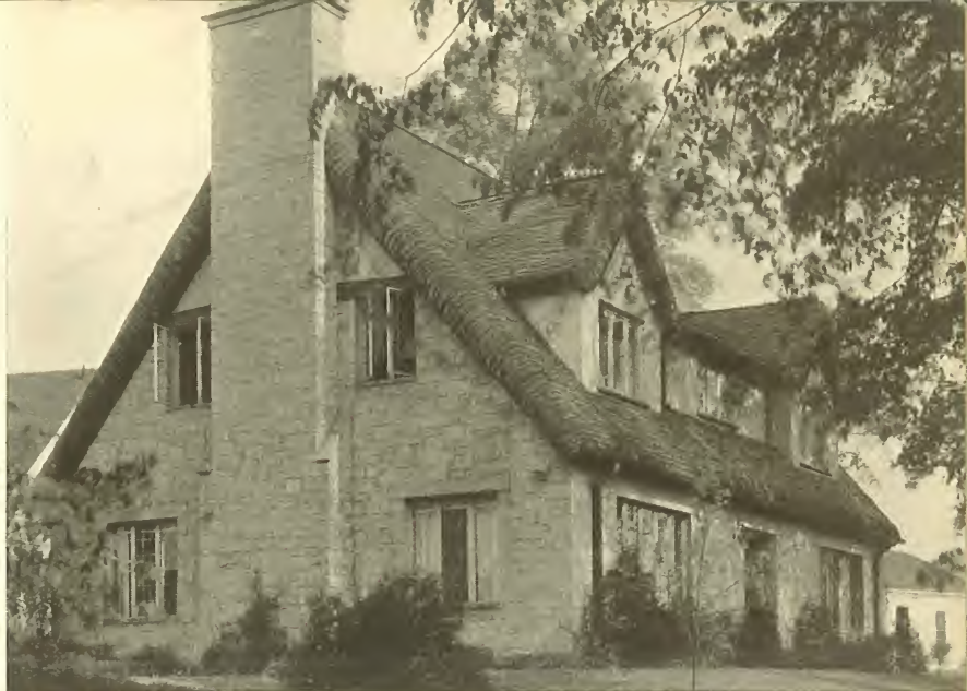
Random ashlar, painted, reveals the attractiveness of concrete masonry for exterior walls. Max Colter, architect, Birmingham, Mich.
